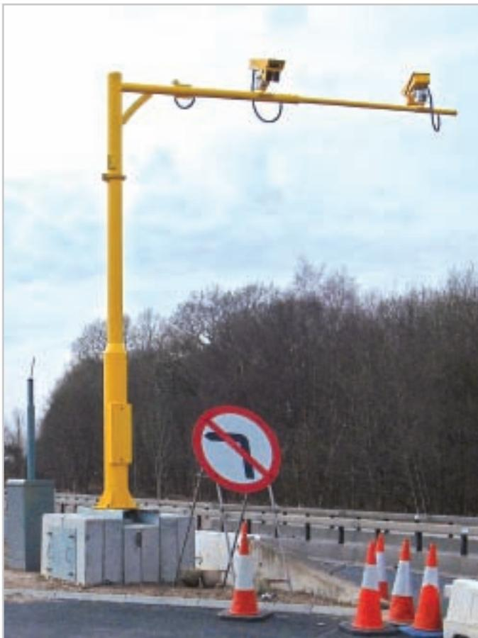
6m cantilever pole with 5m arm
