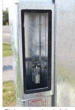
Tilt-down columns have the facility to be padlocked internally
