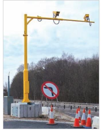
6m cantilever pole with 5m arm
