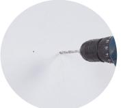
2.Drill the holes on the wall with marked positions
